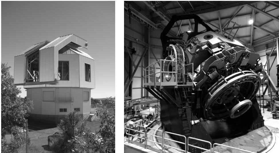
Figure 1. Left: The DCT enclosure. The dome shutter is open, as are the observing level vent doors. The second floor vent doors are the panels just below the bottom of the dome. Right: The DCT Mount.
